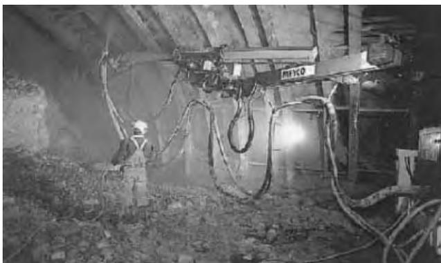
Fig. 1. MEYCO Robojet manipulator.
